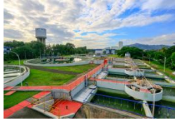
WTP Krenceng 2.000 lps
