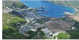
Desal-Demin Water Plant Sumbawa Desal 256 cmh & Demin 65 cmh (Under Construction)
